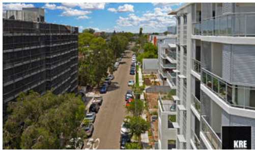
98-100 Railway Terrace, Merrylands
